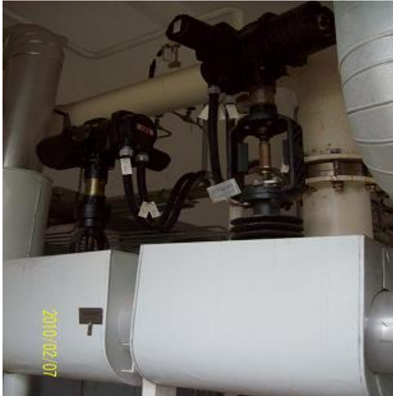
Steam Inlet Control Valve
